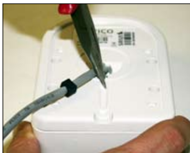
Breaking away the channel stop.
